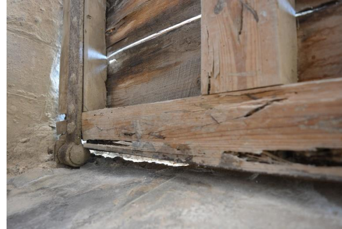
Detall part inferior porta, degradada
